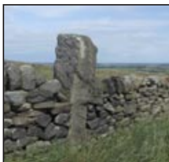
A single stone incorporated into the wall. Bolsterstone Road, Swanheight
